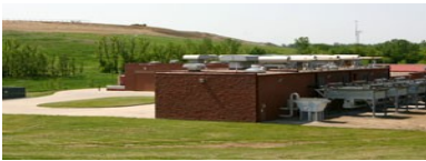
Methane Recover Facility
