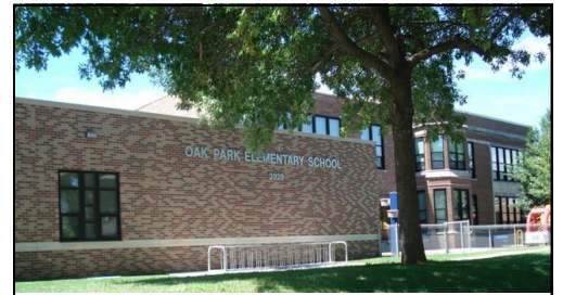
Oak Park Elementary, built in 1891, is the oldest school ENERGY STAR® labeled for 2010, with a current rating of 87.
